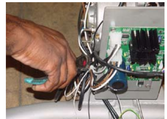
Figure 20 - Cut cable tie
